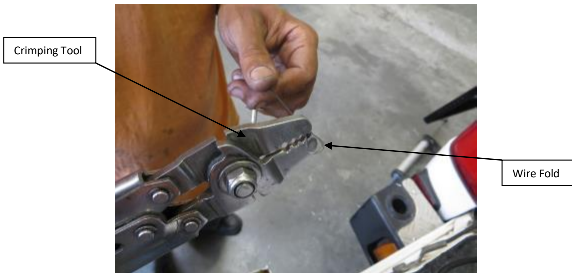
Figure 13: Crimping wires together
