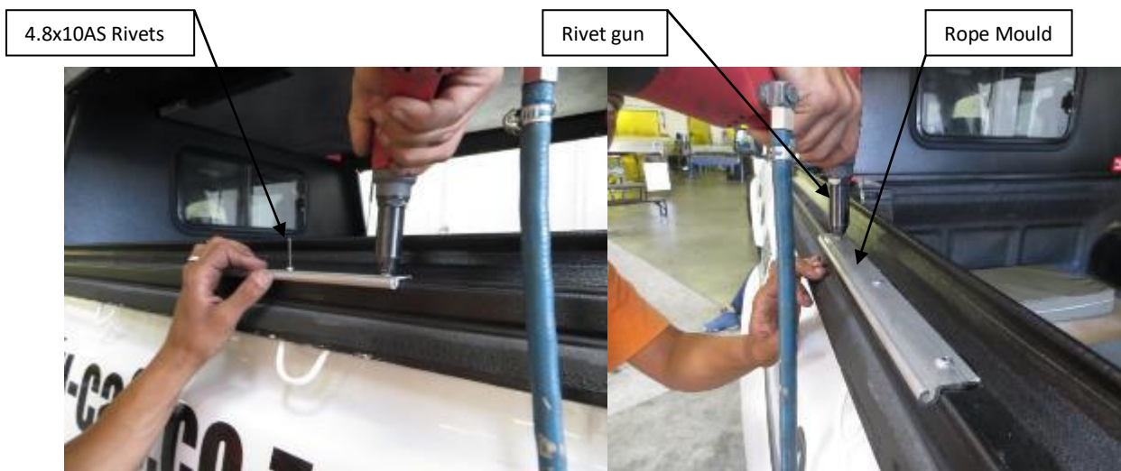
Figure 7: Riveting rope mould to surface
